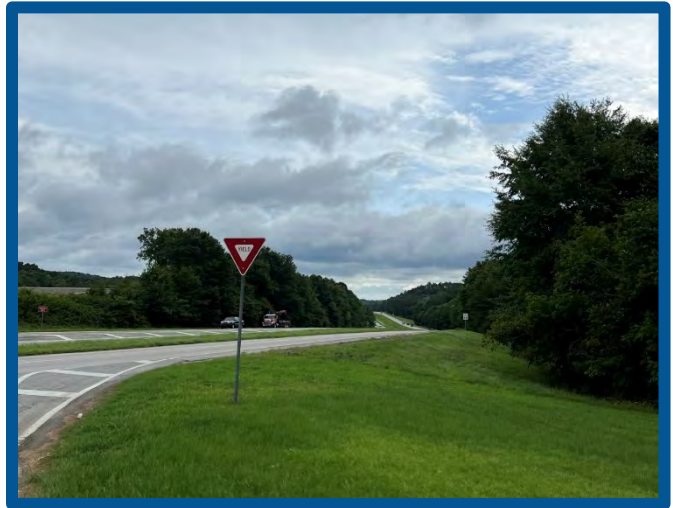
Figure 2-24 Example of Grade Changes on SR 365
