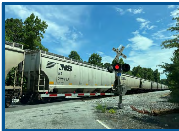
Figure 2-8 At-Grade Railroad Crossing at White Sulphur Road
