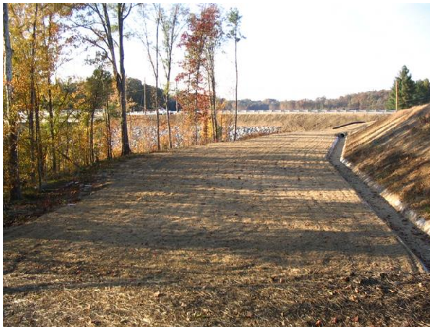
Figure 2.8-6 - Typical level spreader configuration (photo courtesy of NCDOT)
