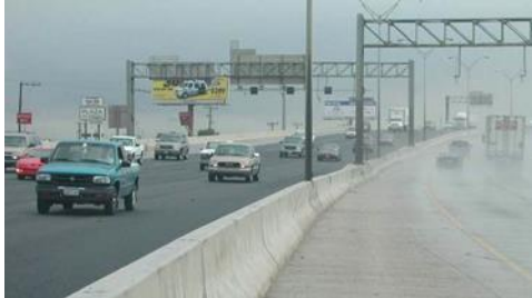
Photo Description: OGFC on Left, Portland Cement Concrete on Right
