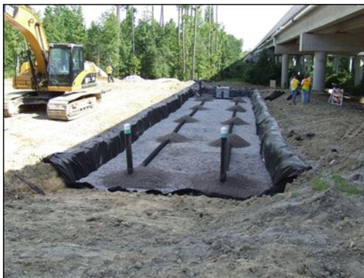
Figure 2.8-4 - Typical underdrain installation (photo courtesy of NCDOT)
