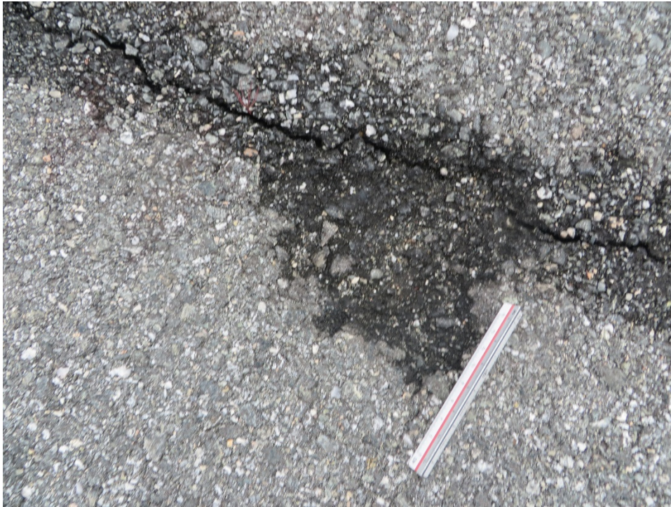
R119NH-10. Raveling (Sample Unit No. 19).
