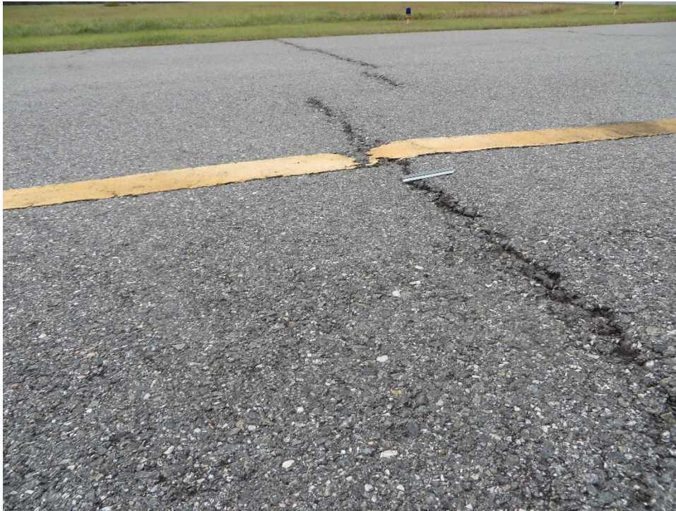
TANH-10. Swelling (Additional Sample Unit No. 01).
