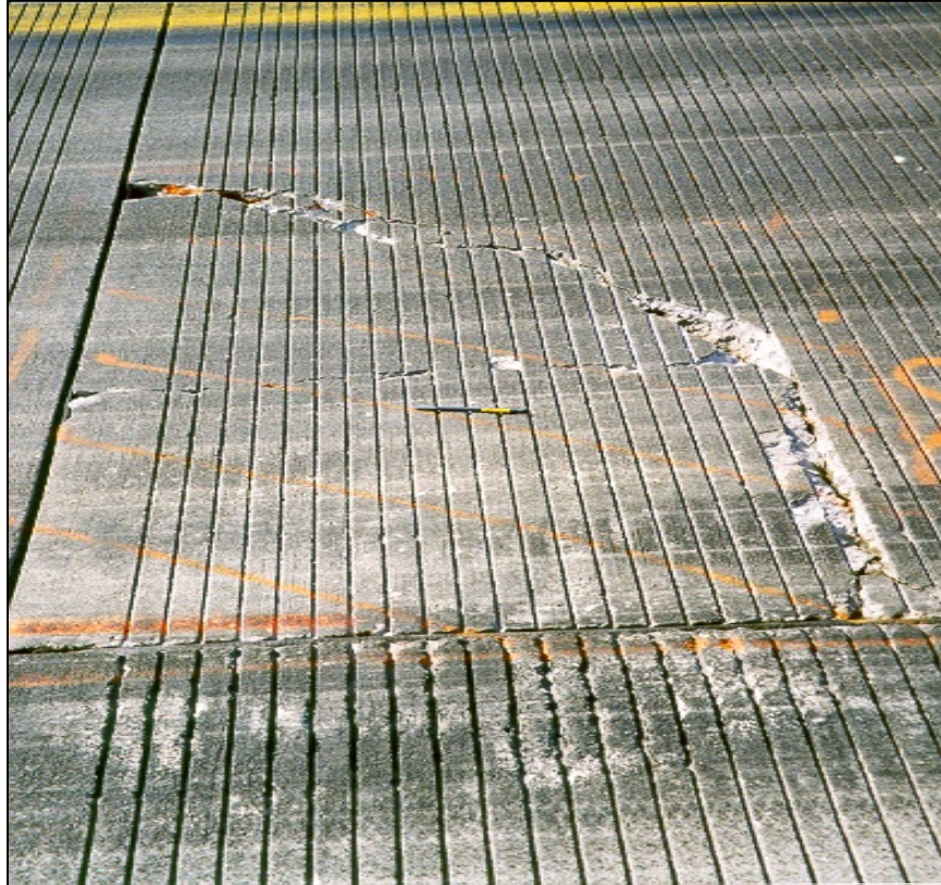
FIGURE H-11 HIGH-SEVERITY CORNER BREAKING
