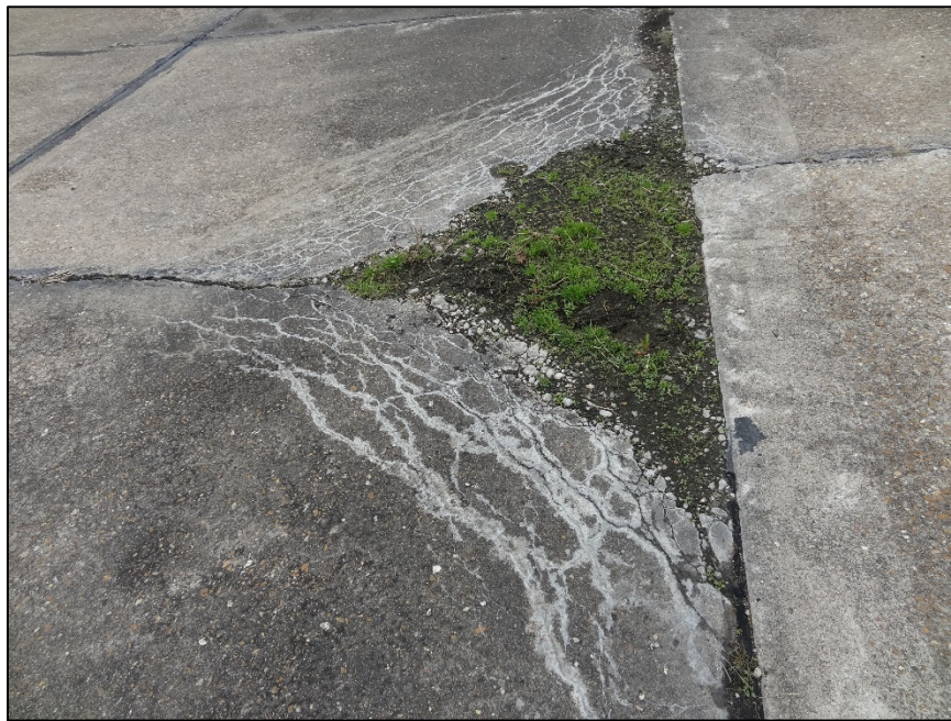
FIGURE H-20 HIGH-SEVERITY ASR
