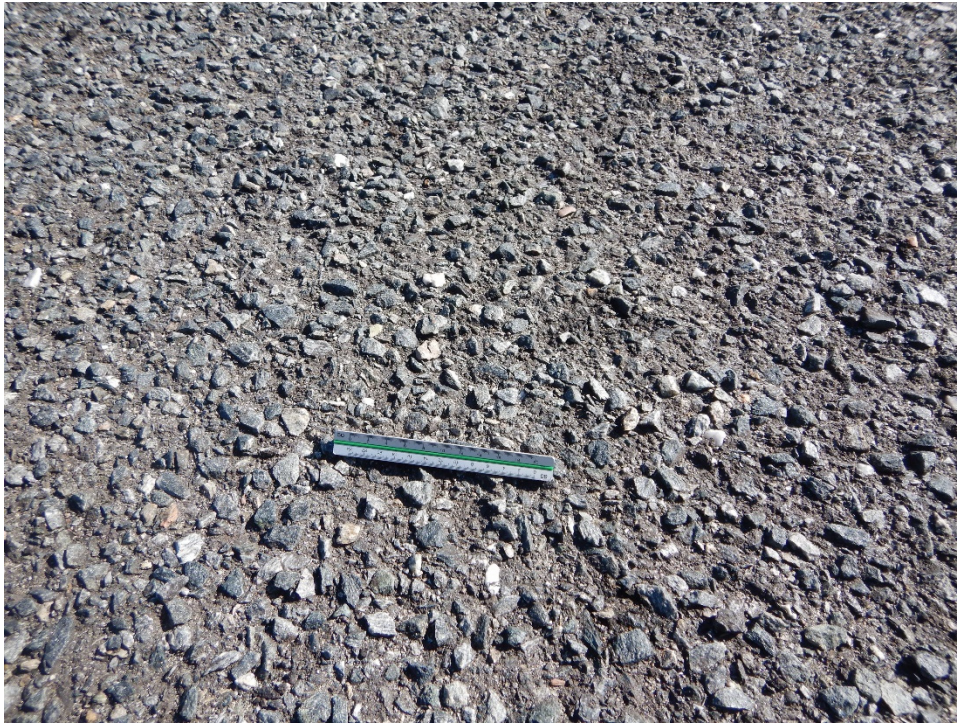
A02BT-10. Raveling (Sample Unit No. 41).
