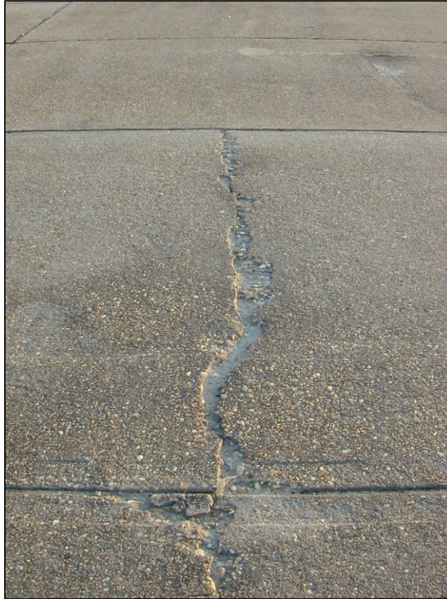
FIGURE H-12 HIGH-SEVERITY LTD CRACKING
