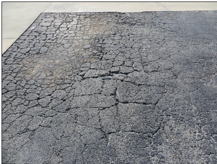
FIGURE H-1 HIGH-SEVERITY ALLIGATOR CRACKING
