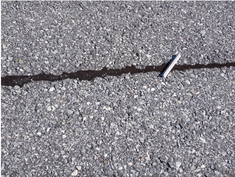
R119BT-20. L&T Cracking (Sample Unit No. 04).
