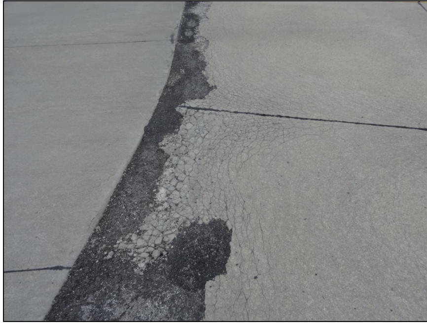
FIGURE H-13 HIGH-SEVERITY DURABILITY CRACKING
