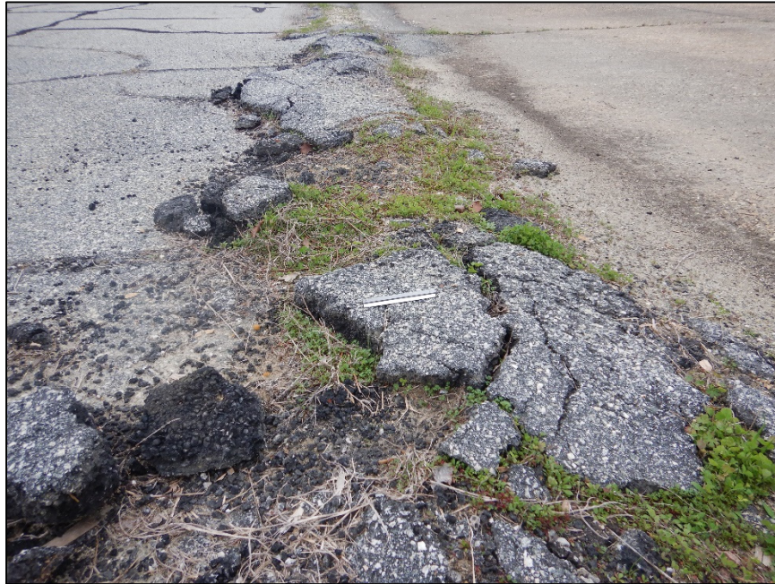
FIGURE H-8 HIGH-SEVERITY SHOVING AT AC/PCC INTERFACE
