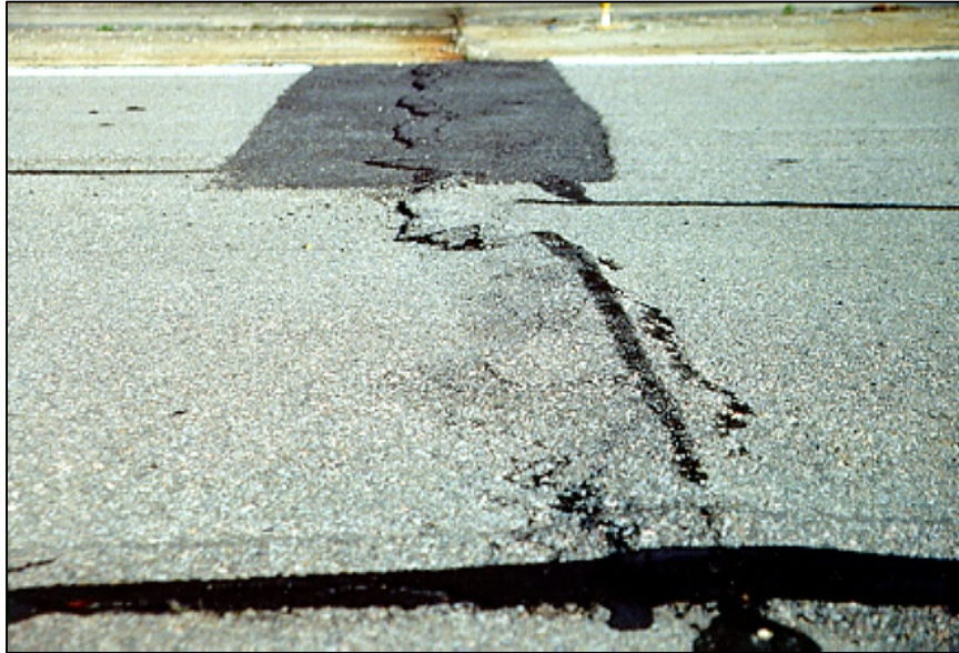
FIGURE H-9 HIGH-SEVERITY SWELLING
