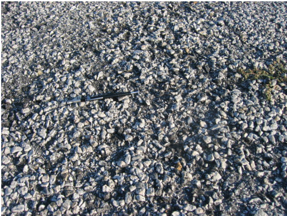
A01GF-20. Raveling and weathering.
