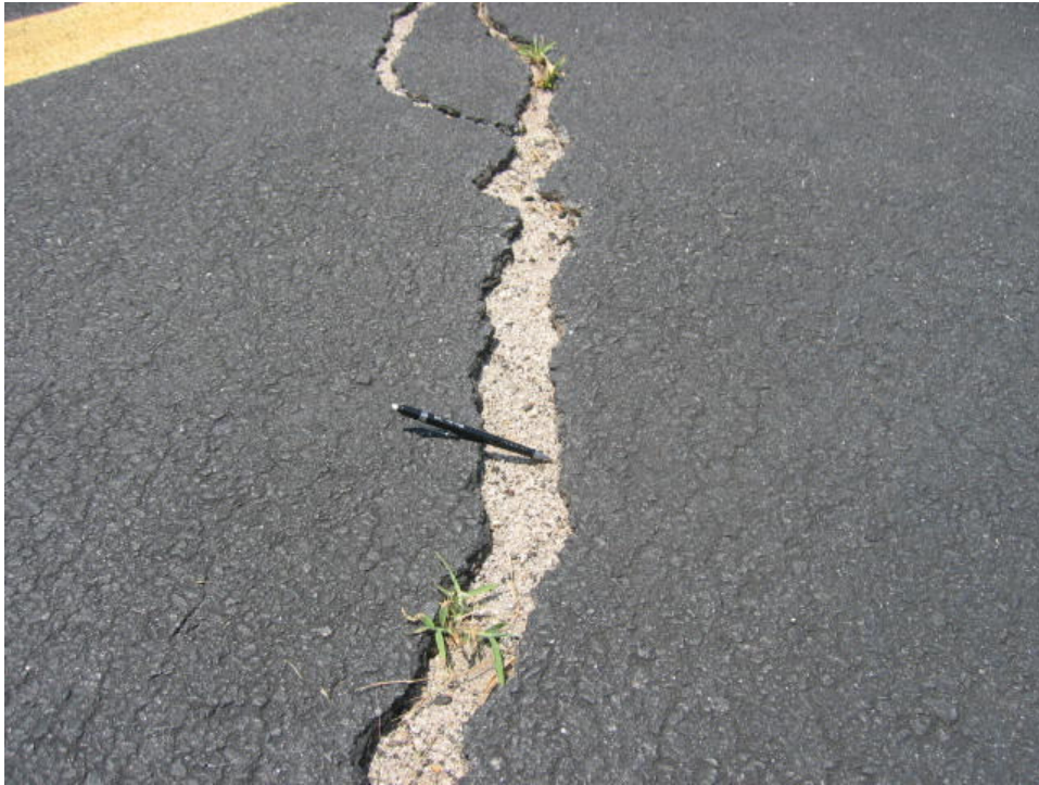
A02GF-20. L&T cracking.
