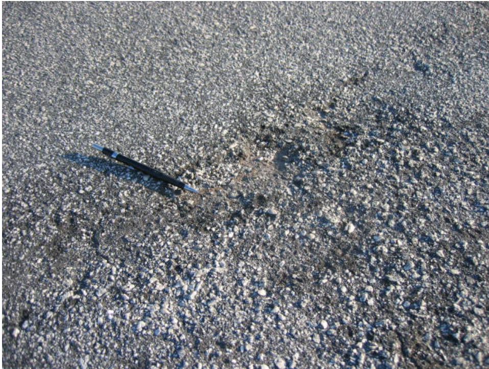
A01GF-10. Raveling and weathering.
