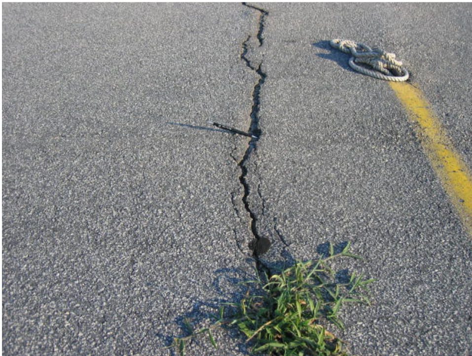
A01GF-10. L&T cracking.
