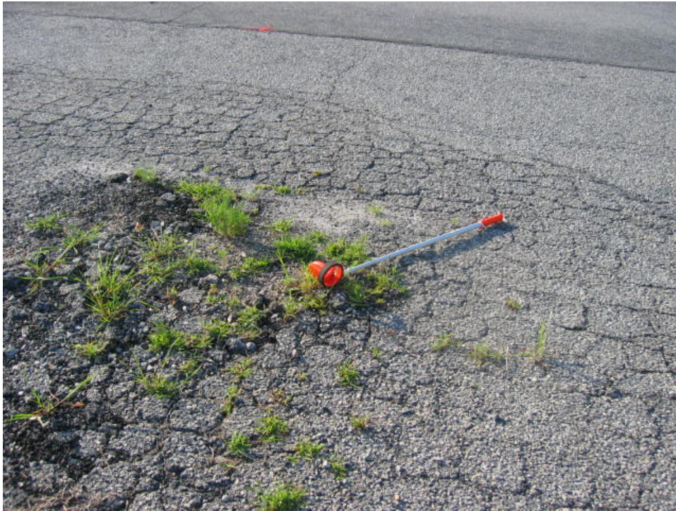
A01GF-20. Alligator cracking.
