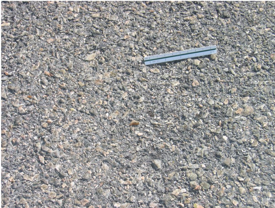
R119NH-10. Raveling and weathering.
