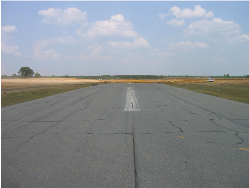
R523CH-10. Overview (new construction).
