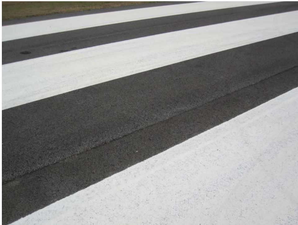
R119NH-10. Satisfactory Paint.
