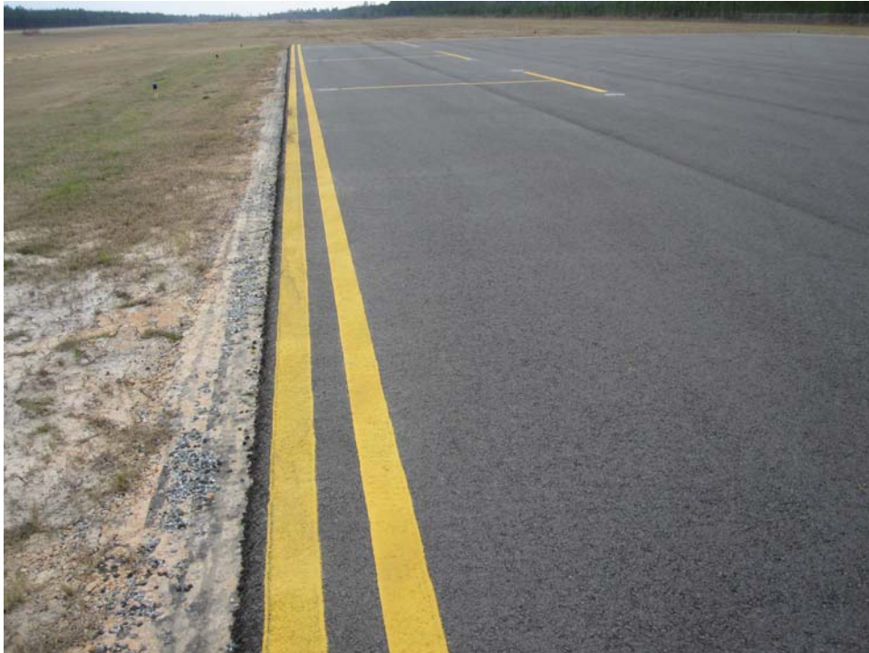
A01NH-10. Satisfactory Paint.
