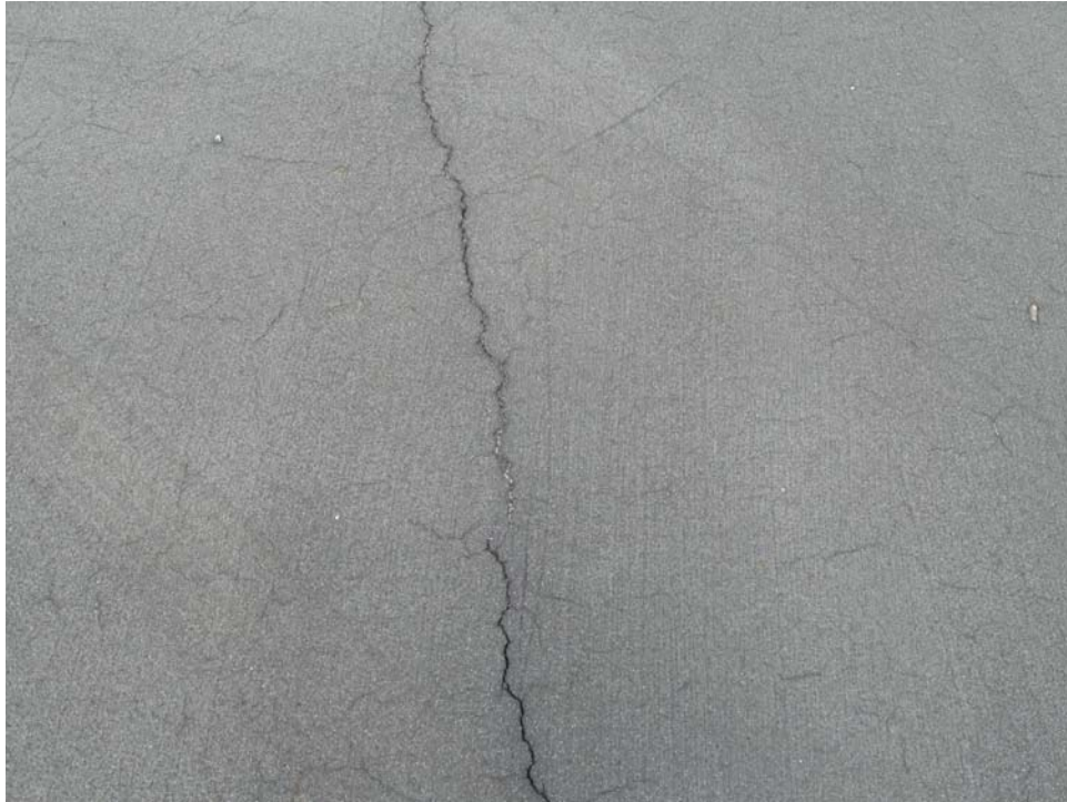
A02GF-50. Longitudinal and Transverse Cracking (Sample Unit #01).
