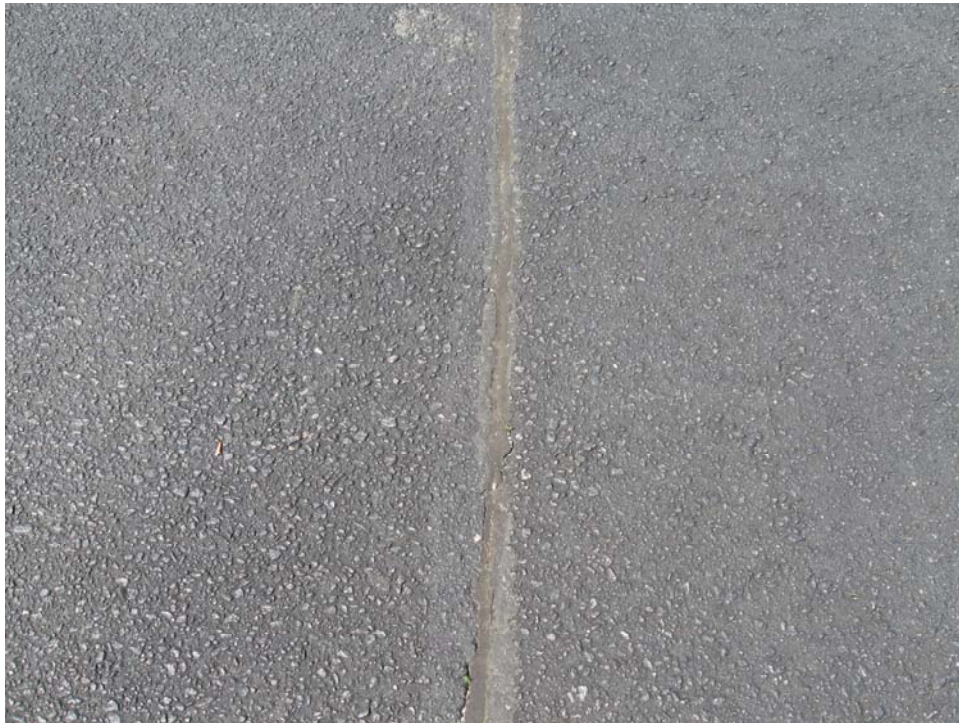
TH01GF-10. Longitudinal and Transverse Cracking (Sample Unit #09).
