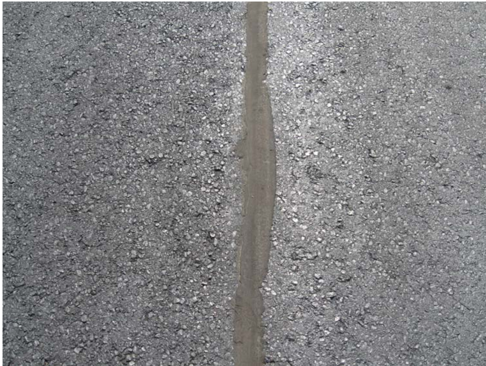
TBGF-10. Longitudinal and Transverse Cracking (Sample Unit #04).
