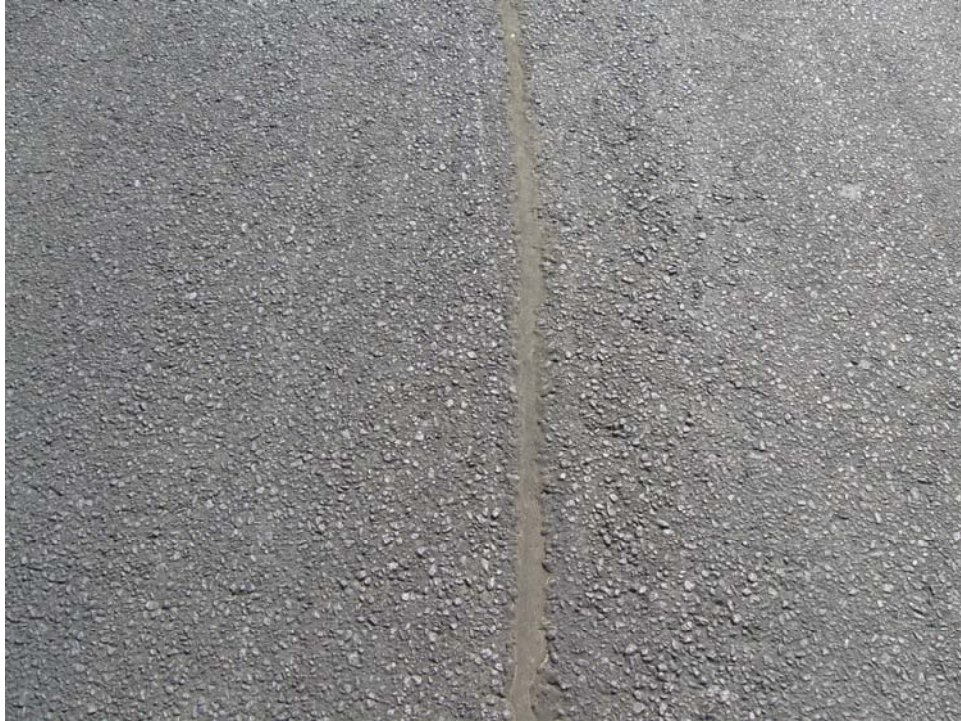
TBGF-40. Longitudinal and Transverse Cracking (Sample Unit #02).
