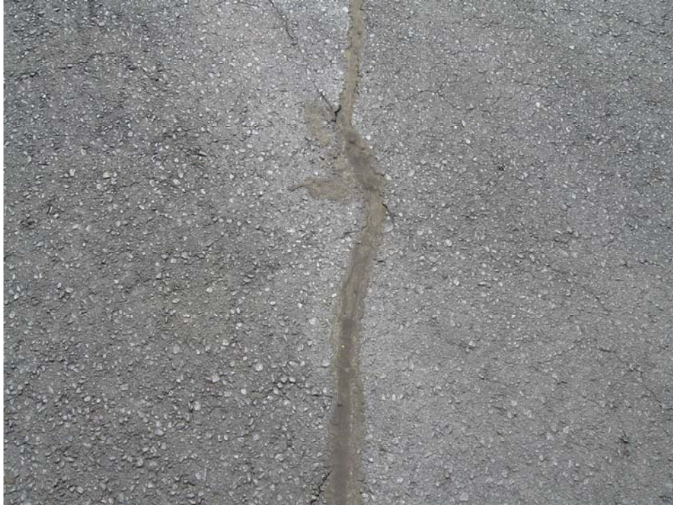
A02GF-60. Longitudinal and Transverse Cracking (Sample Unit #01).
