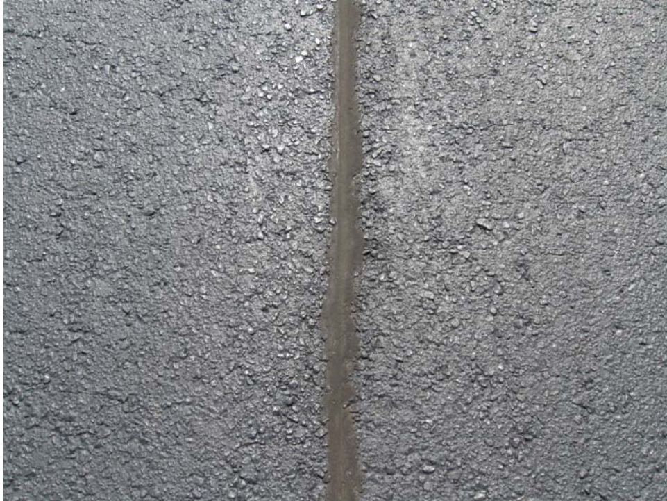
TBGF-20. Longitudinal and Transverse Cracking (Sample Unit #05).
