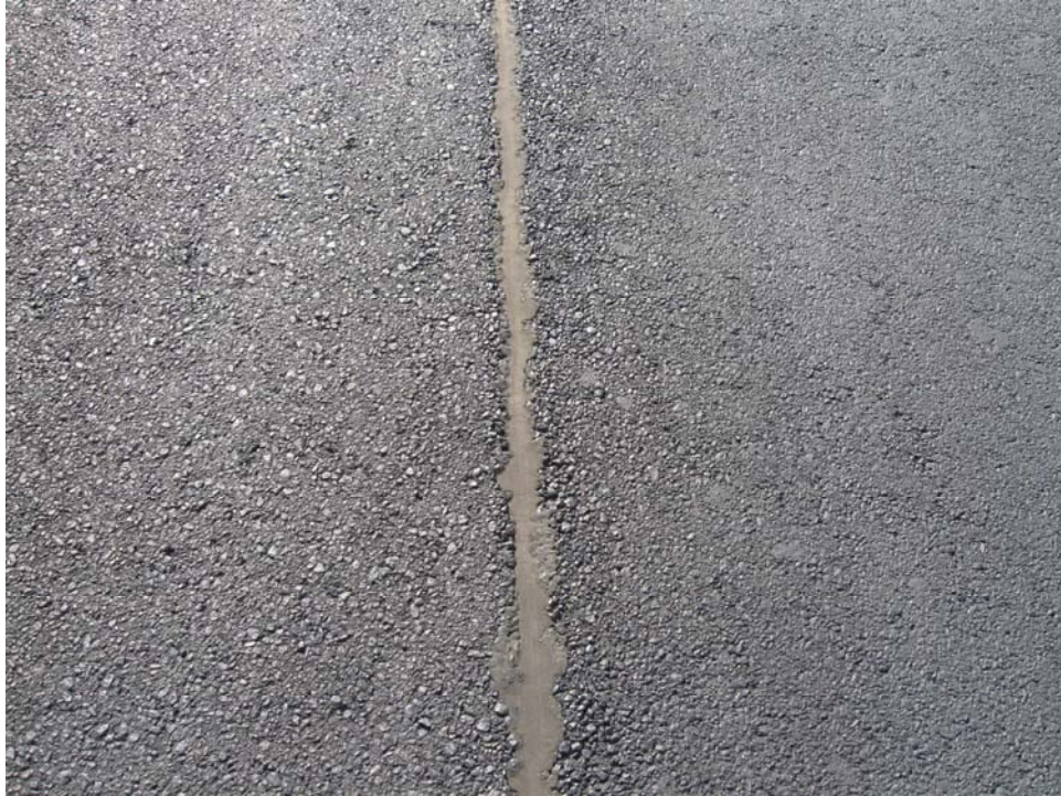
TAGF-10. Longitudinal and Transverse Cracking (Sample Unit #04).
