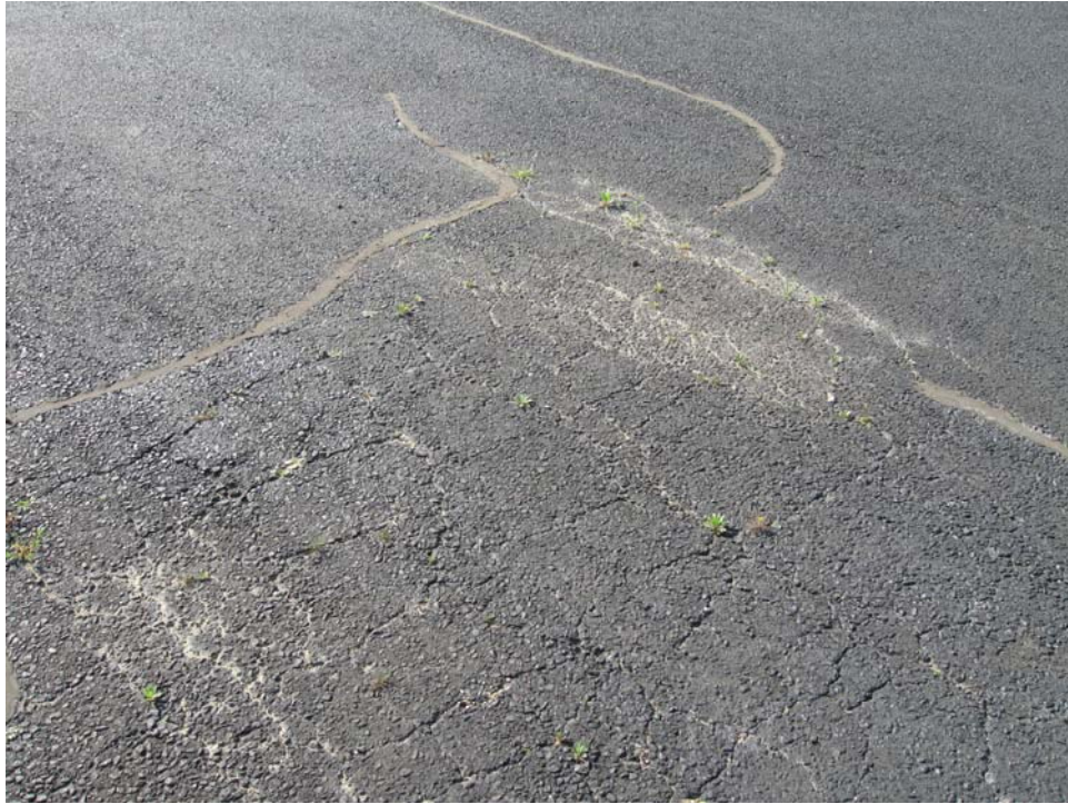
A01GF-20. Alligator Cracking (Sample Unit #02).
