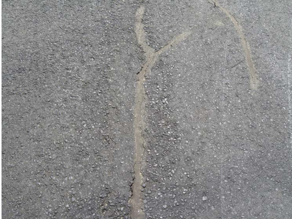
A02GF-40. Longitudinal and Transverse Cracking (Sample Unit #01).
