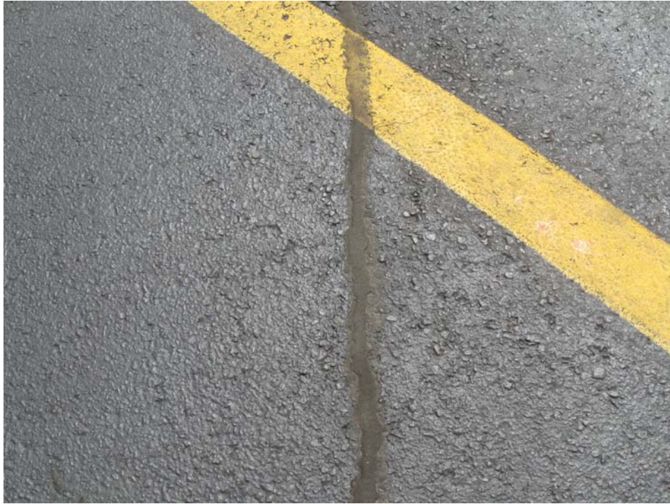
A02GF-20. Longitudinal and Transverse Cracking (Sample Unit #12).
