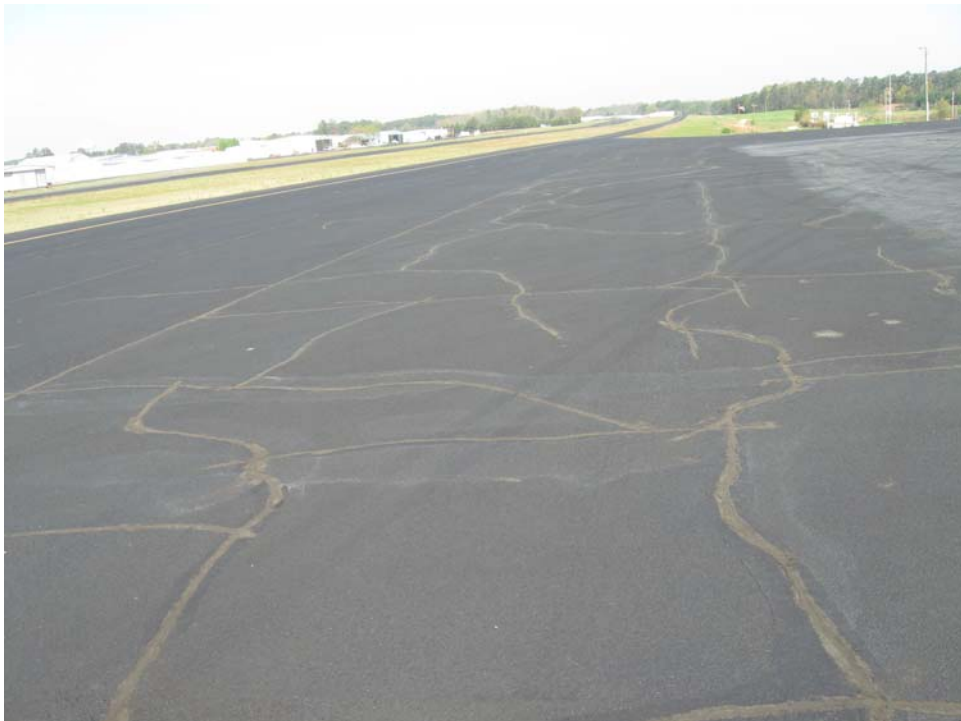
A01GF-10. Block Cracking (Sample Unit #03).
