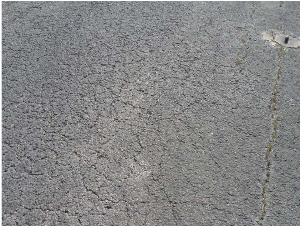
A02GF-30. Alligator Cracking (Sample Unit #01).
