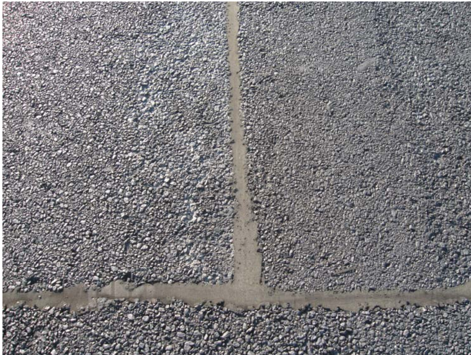
R1432GF-10. Longitudinal and Transverse Cracking (Sample Unit #02).
