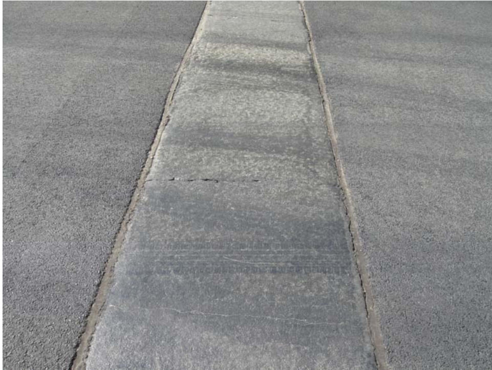
A02GF-70. Patching (Sample Unit #10).
