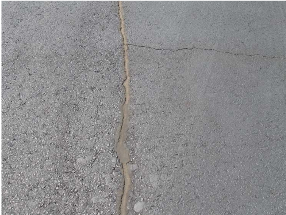
A02GF-10. Longitudinal and Transverse Cracking (Sample Unit #12).
