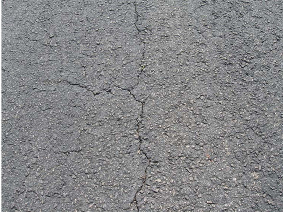
TBGF-30. Longitudinal and Transverse Cracking (Sample Unit #03).
