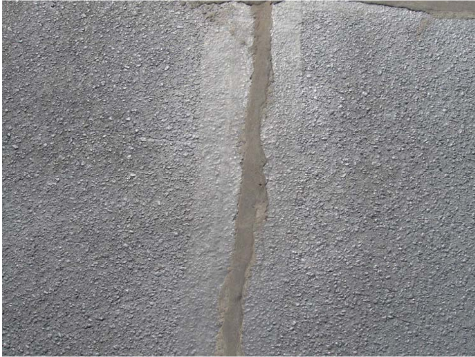
A01GF-10. Longitudinal and Transverse Cracking (Sample Unit #03).
