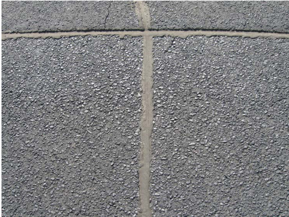
A01GF-20. Longitudinal and Transverse Cracking (Sample Unit #03).
