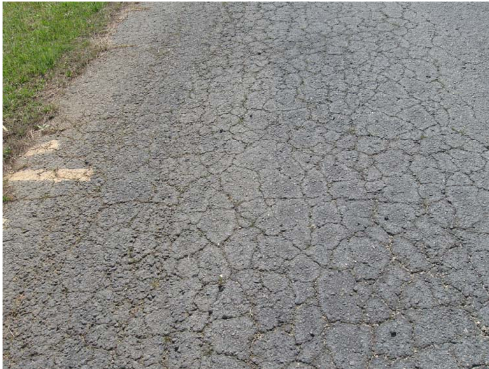
TBGF-30. Alligator Cracking (Sample Unit #03).
