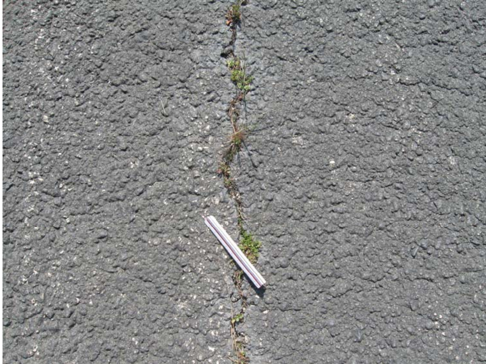
A02GF-30. Longitudinal and Transverse Cracking (Sample Unit #01).
