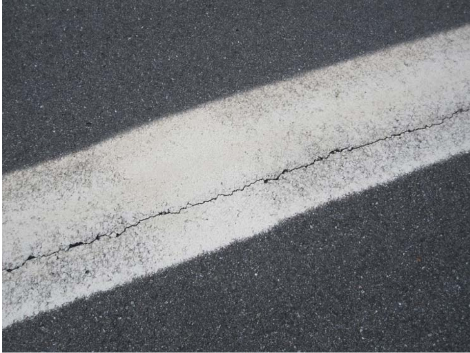
R1129CH-10. Satisfactory Paint.
