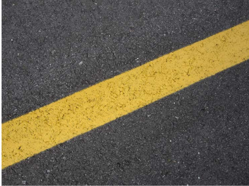
TACH-20. Satisfactory Paint.
