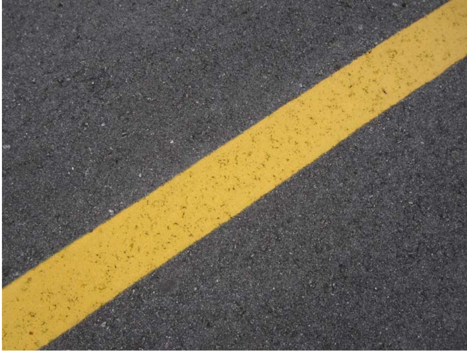
TACH-30. Satisfactory Paint.
