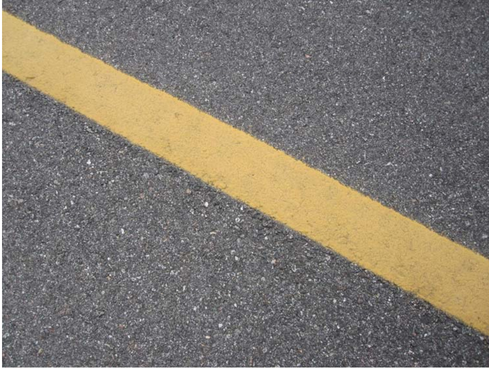
TBCH-10. Satisfactory Paint.
