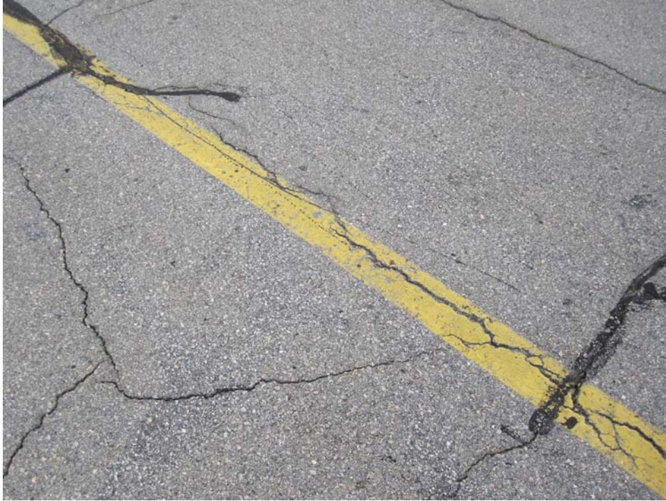
TACH-10. Unsatisfactory Paint.
