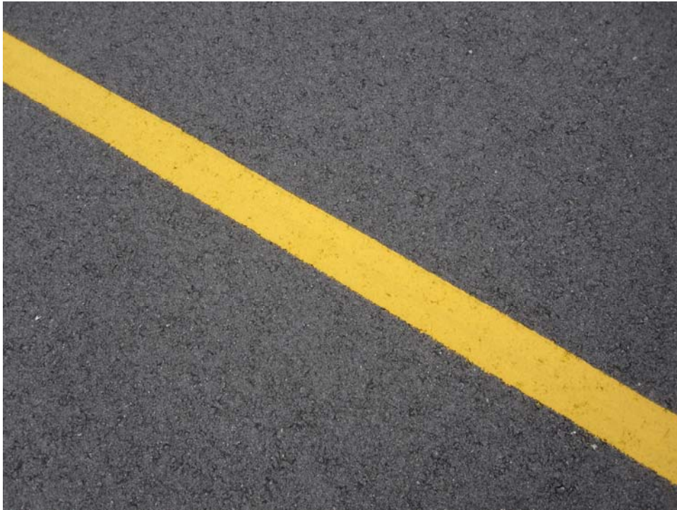
A01CH-20. Satisfactory Paint.
