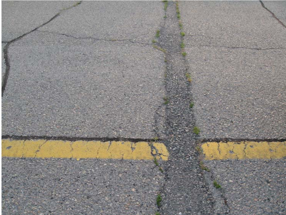
TABT-10. Longitudinal and Transverse Cracking (Sample Unit #04).
