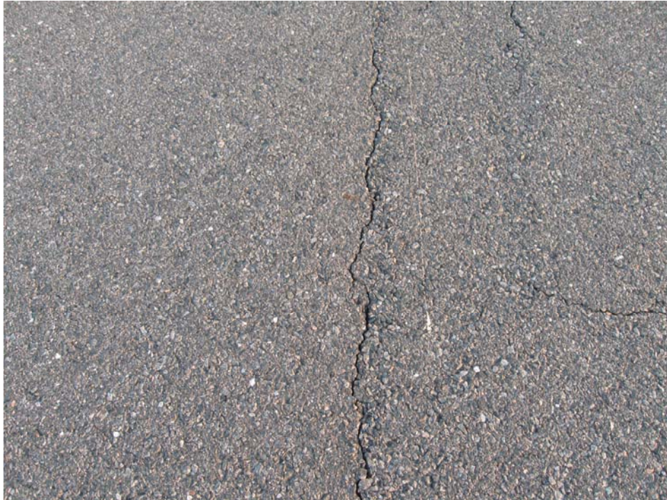
R1836BT-10. Longitudinal and Transverse Cracking (Sample Unit #03).
