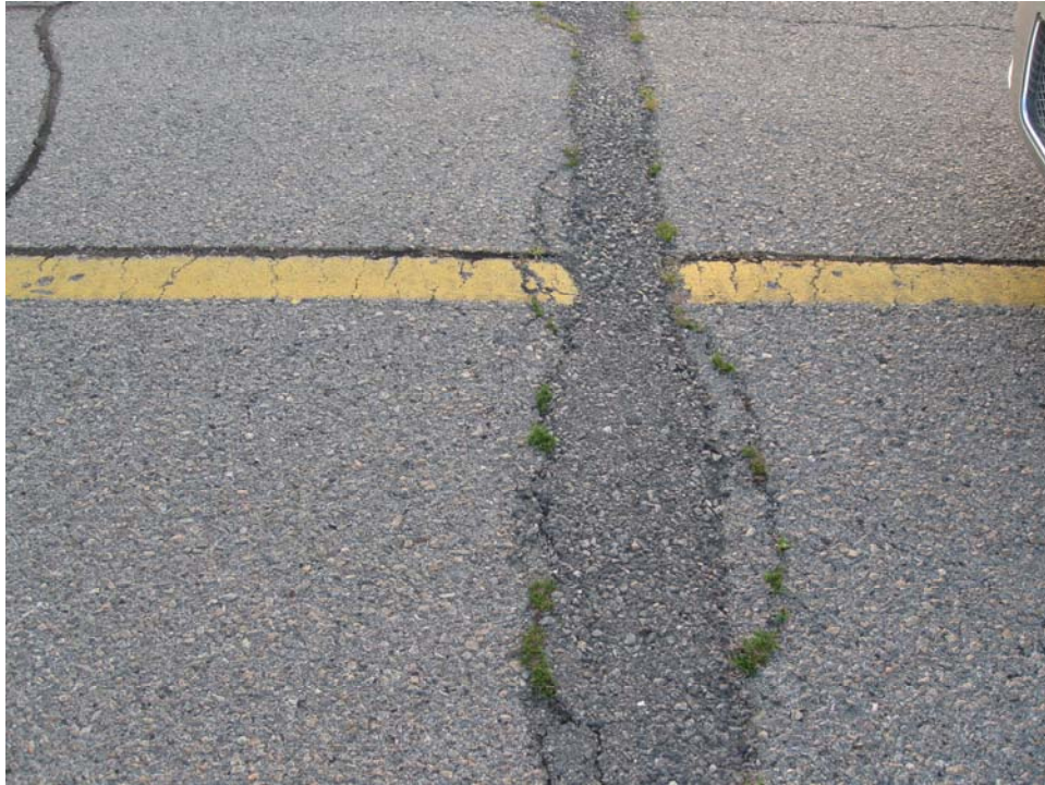
TABT-10. Patching (Sample Unit #04).
