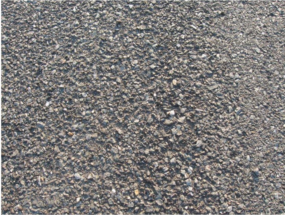
A02BT-10. Raveling (Sample Unit #04).
