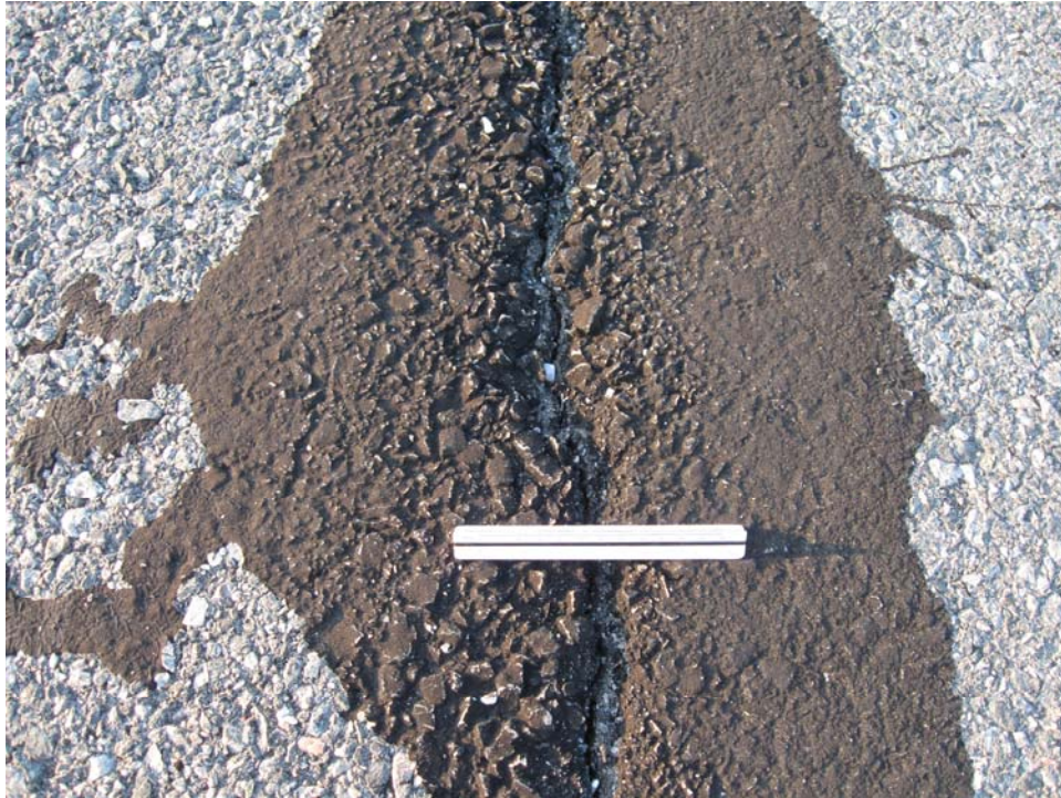
R1836BT-10. Longitudinal and Transverse Cracking (Sample Unit #28).
