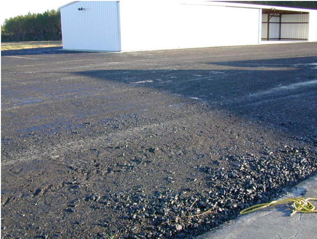
Overview of section THANGJS-10 (new construction).
