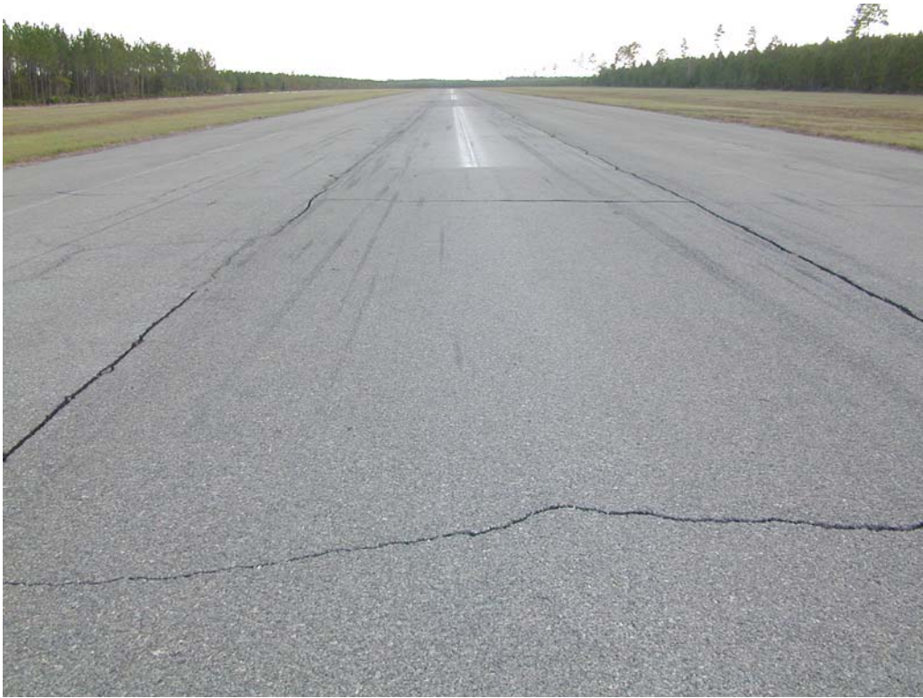
Overview of section R119NH-10.
