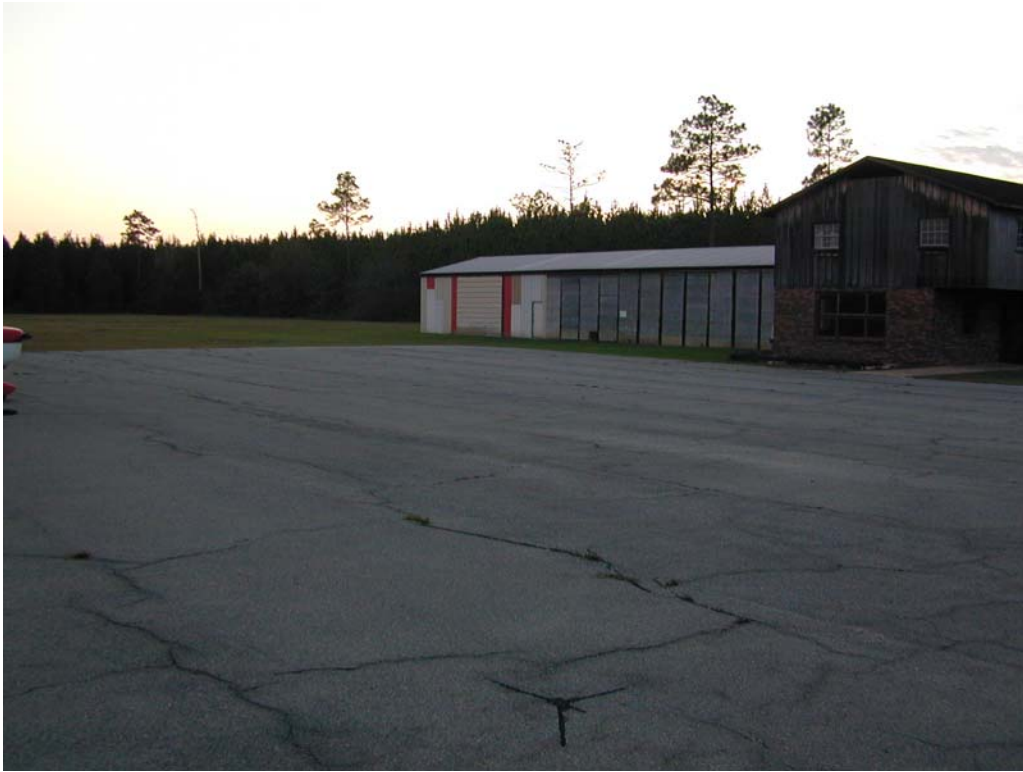
Overview of section A01NH-10.
