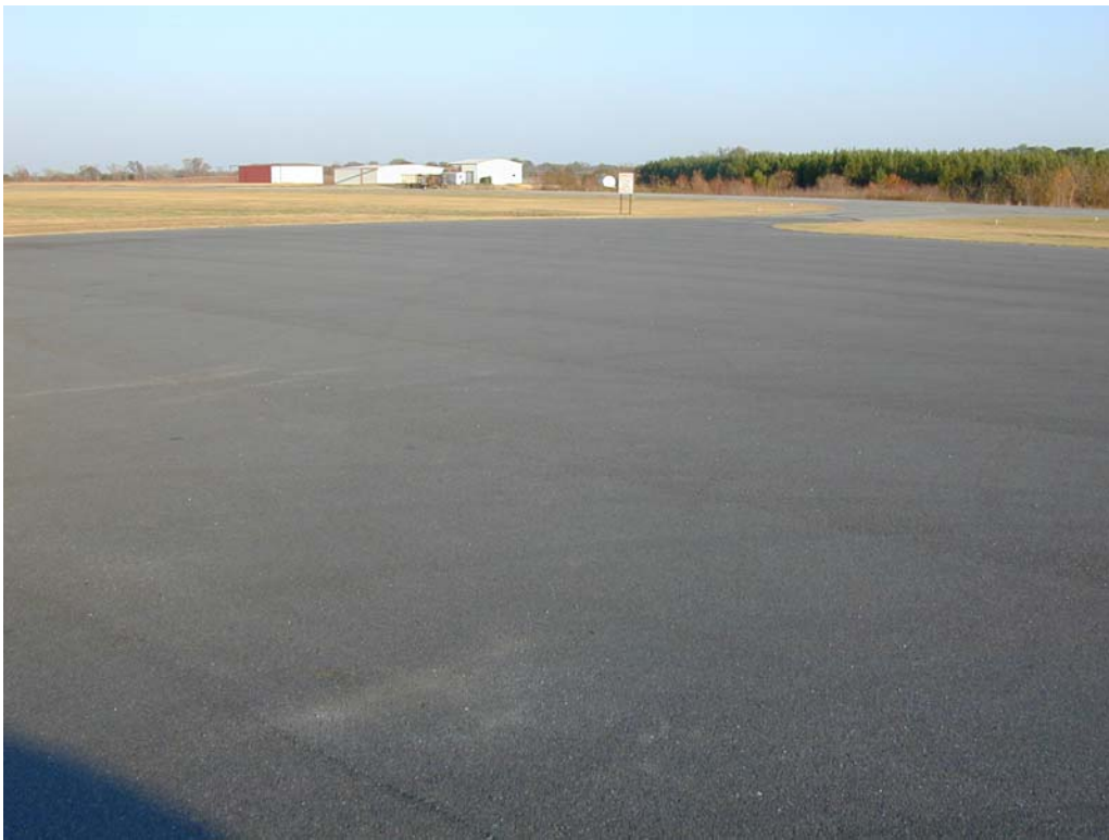
Overview of section A01CH-10.
