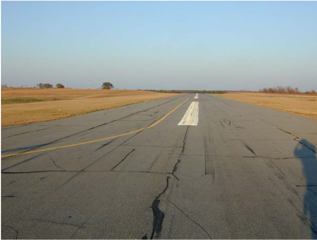
Overview of section R523CH-10.
