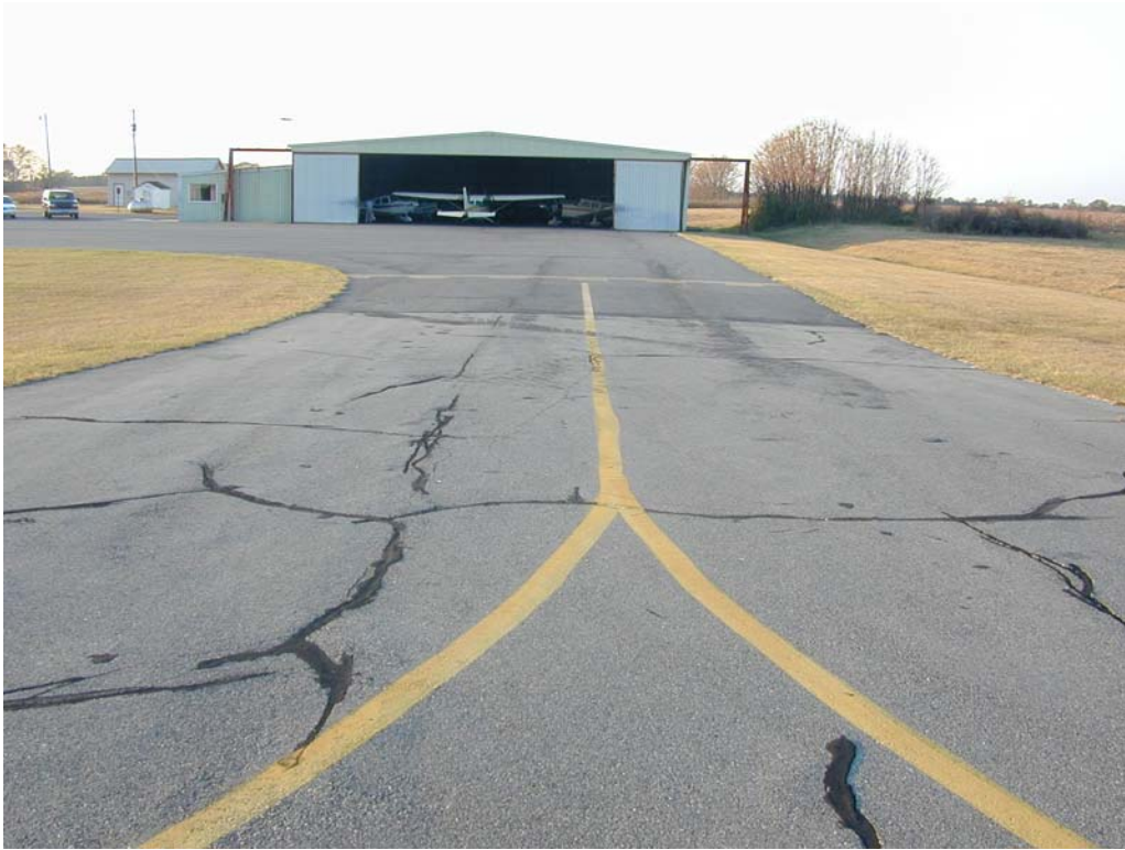
Overview of section TACH-10.
