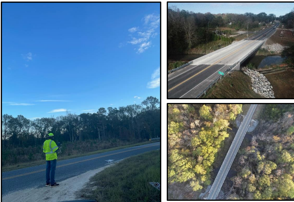
PI 0013942 – SR 1(US 27) over Long Cane Creek – Troup Co PI 0016804 – Lowery Firehouse Road over Ochwalkee Creek – Laurens Co PI 0017311 – Piney Grove Road over Colemans Creek – Appling Co Images taken by UAS Pilot Robert “Greg” Ellison
