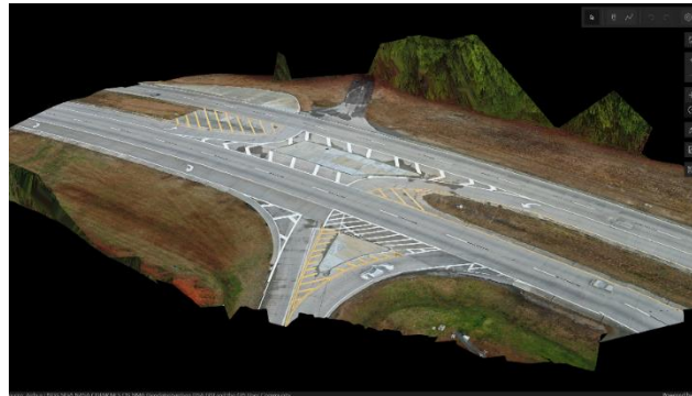
QR Project S015821, SR 316 at Williams Farm Road, RCUT. The project aims to reduce potential crash points and improve traffic flow on major roads. UAS Mission flown by Demario Hall. Visual Observer, Lewis Brooker
