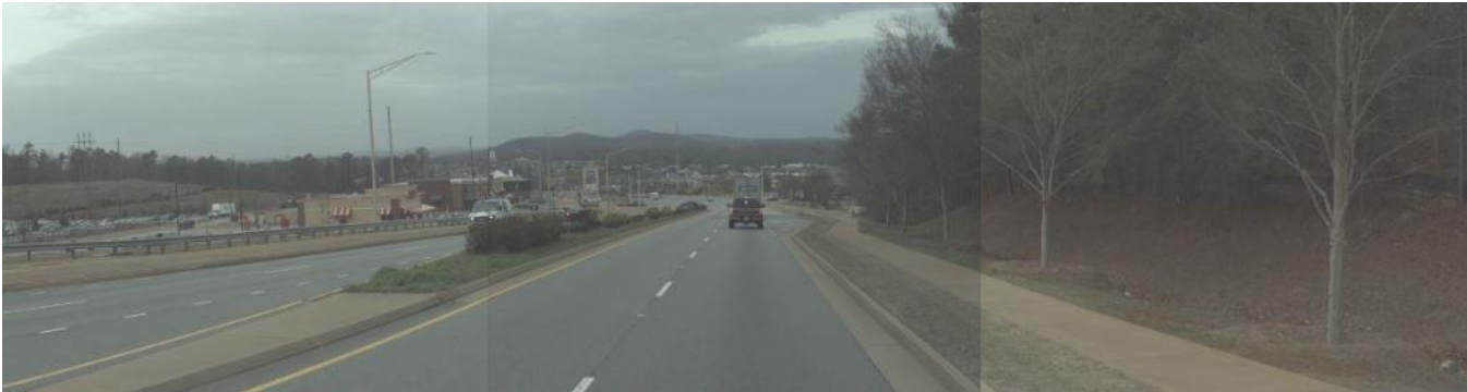
A Mainline Road in Bartow County, State Route 113 westbound, in the decreasing Milepoint Direction
