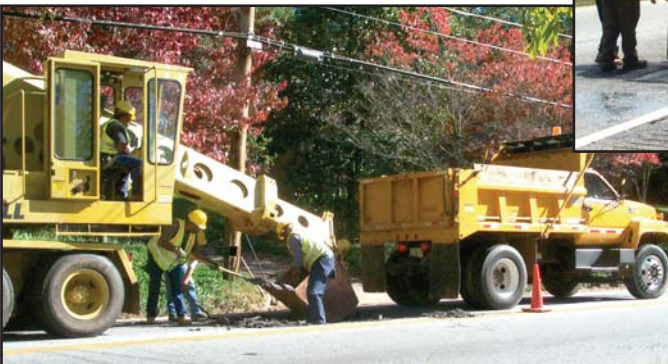
Maintenance Area 5 performs deep-base patching.
