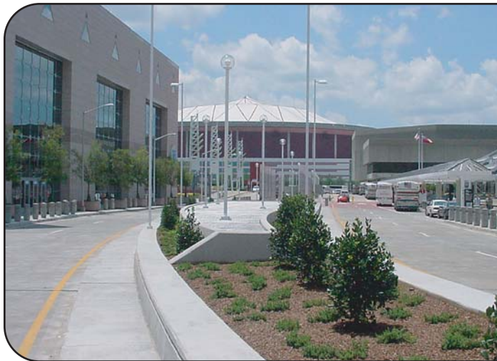
Construction was completed at Andrew Young International Boulevard during the fiscal year
