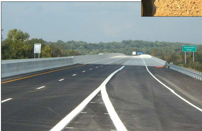
Construction along Interstate 520 (Bobby Jones Expressway Extension) was completed in FY 2004.
