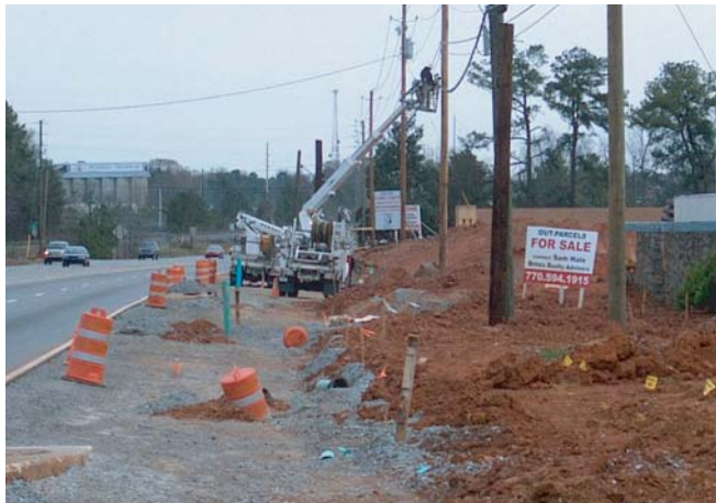
The Office of Utilities performs utility relocations.
