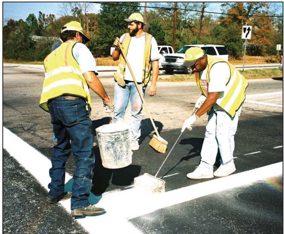
Maintenance crew cleaning and painting road in District One.
