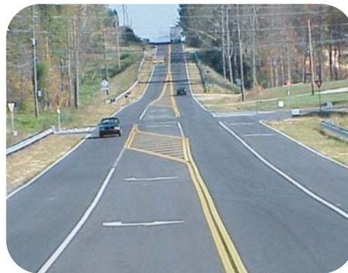
State Route 20- widening and reconstruction project in Floyd County
