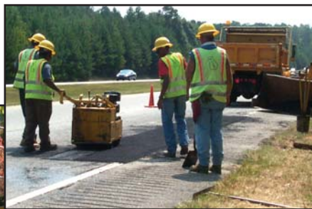
Pavement patching on SR 74 in Fayette County
