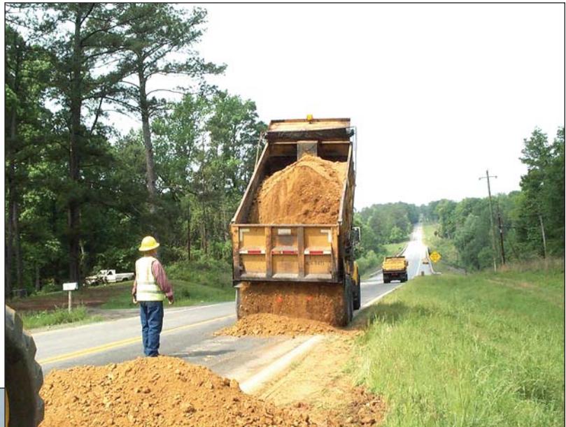
District Two Maintenance employees rebuild shoulder.
