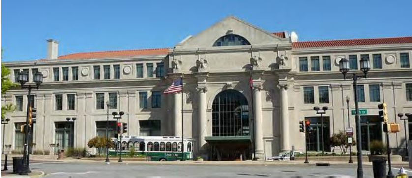
Figure 40: Terminal Station - Macon, GA
